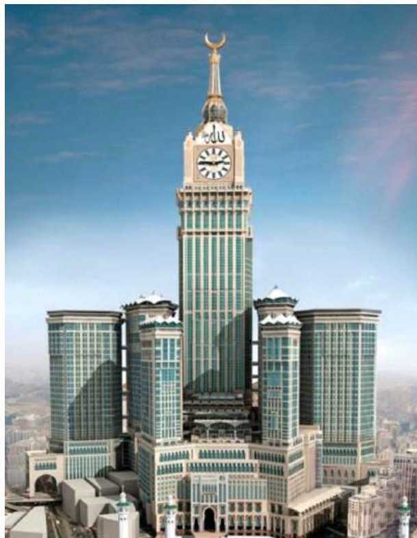
Mekkah Clock Tower, Mecca
