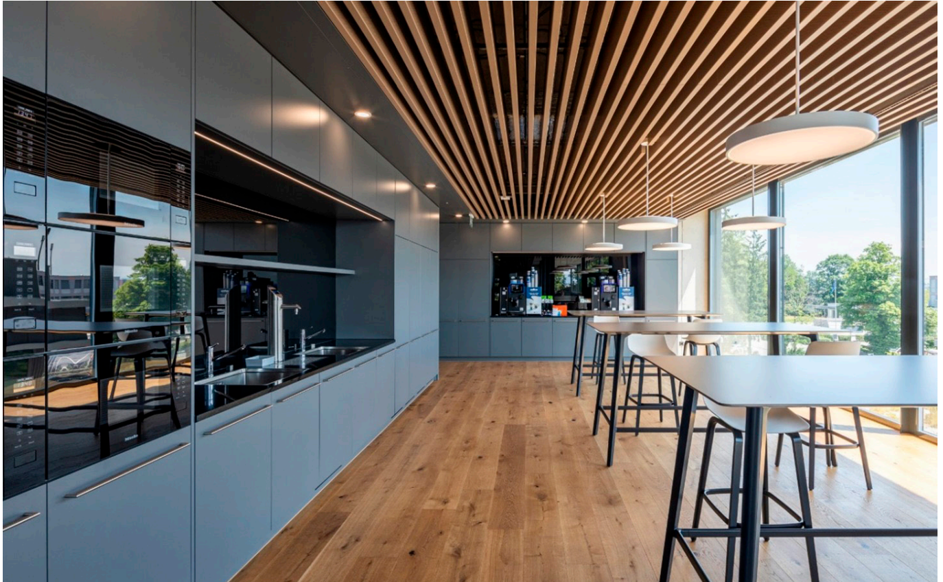
Fig. 10: Baffles constitute a suitable shape for ceiling absorbers. The image shows heating/cooling baffles with an additional layer of sound absorption material (acoustic fleece and mineral wool mats).
