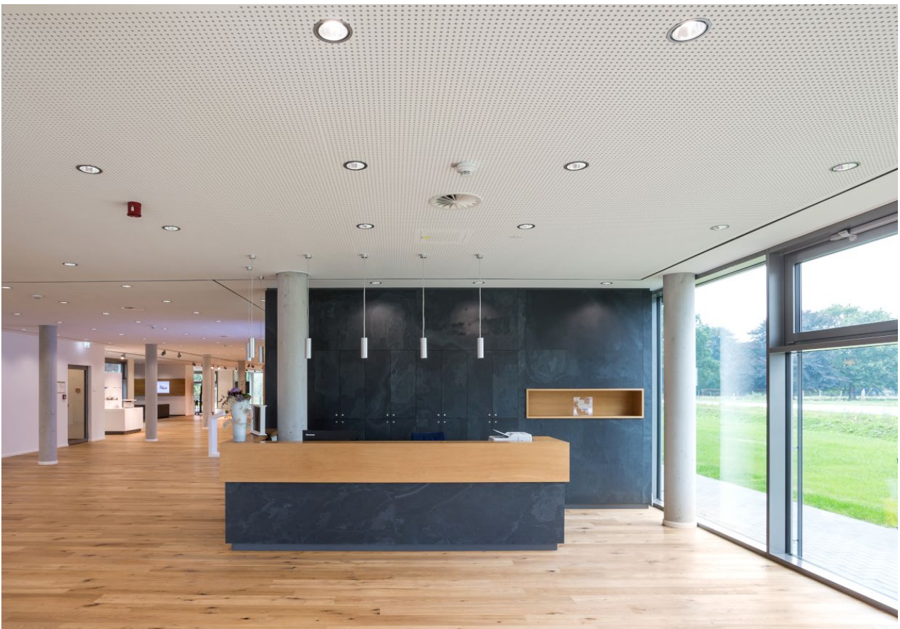
Fig. 7: Radiant ceiling with perforated plasterboard panels and different fixtures (light, air, sprinkler, smoke detector)
