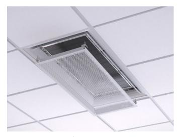
Figure 12. Removing the face plate to access the coil
